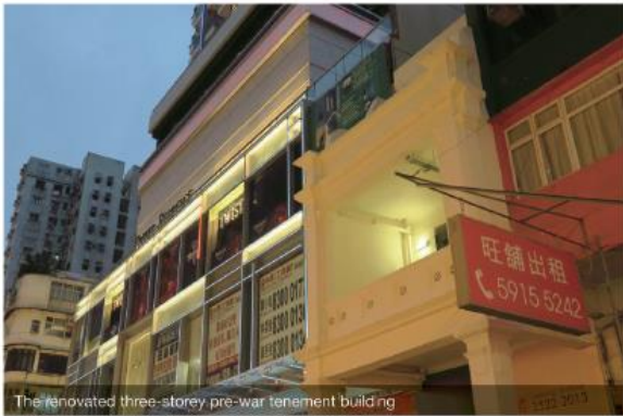
The renovated three-storey pre-war tenement building
