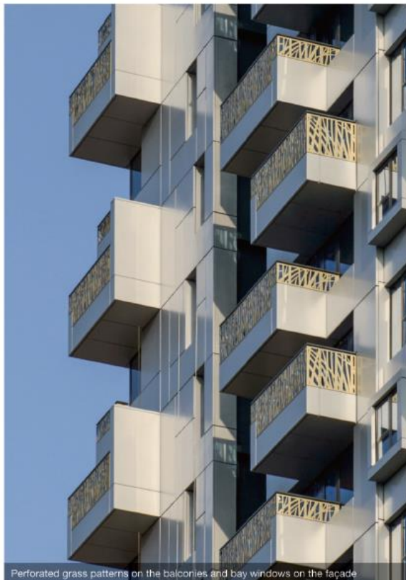
Perforated grass patterns on the balconies and bay windows on the façade
