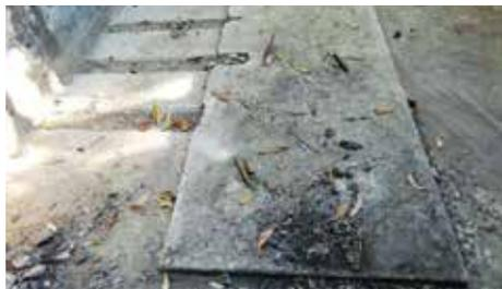
**Figure 83:** The engine platform and cable ducts. Metal plating originally covered the ducts to protect the power cables below. Note the long bolts used to install the engine on platform (photo by author in 2019).
