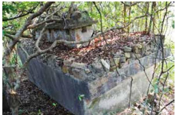
Figure 20: Roof of the toilet shelter camouflaged by rocks and earth. Three ventilation shafts on top typified pit toilet shelters (photo by author, 2015).
