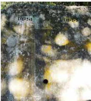
**Figure 84:** The rear wall inside with open hole for pipeline. Bricks embedded at top of wall have holes for ventilation (photo by author in 2019).
