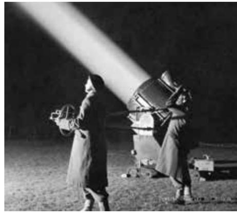
**Figure 4:** A 90 cm searchlight with tracked wheels in operation during WWII. Note the operator using an extended control arm to maintain distance from the light (Imperial War Museum collection).
