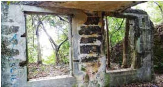
**Figure 69:** Inside of the front wall and window of the store room. The square hole at the top right is for ventilation (photo by author in 2014).
