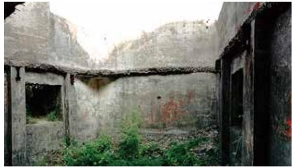
**Figure 38:** The front of the Tai Leng Tung AOP from the inside. Two large I-beams were used to support the upper level structure. Two windows were on the lower level used for large equipment installation and ventilation. Two trenches connected to these windows separately (photo by author in 2016).
