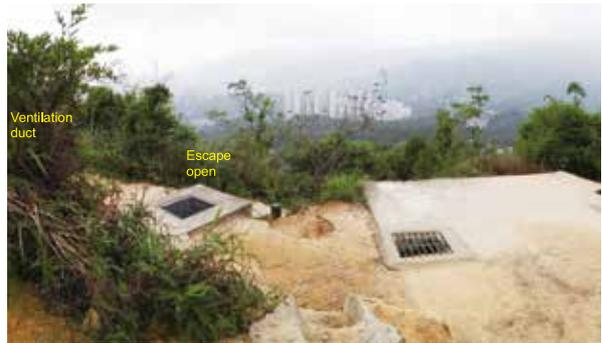
**Figure 23:** Roof of the Shing Mun AOP. An opening on the AOP's roof was caused by scavengers removing steel reinforced bars from the supporting beam (photo by author in 2014).
