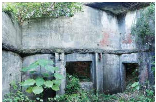
Figure 46: The right interior of the Ping Tok Hang Shan AOP. Its design was the same as that of the Tai Leng Tung AOP. The roof and upper floor of this AOP were demolished after the war (photo by author in 2016).
