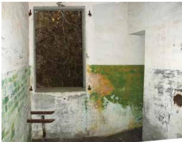
**Figure 19:** The kitchen with rack and pipe for a basin on the left. The hole in the wall on the right is a chimney for the stove. The opening on the right leads to a storeroom. The window had steel shutters before (photo by author in 2005).
