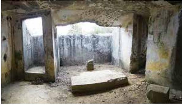
**Figure 25:** The front of the Shing Mun AOP from the inside. The field artillery scope position was on its left-hand side. The DPF was on its right with a large concrete platform in the back. The three concrete blocks supported the DPF, but two have collapsed and only one remained in its original position. Note the battle damage on the roof and an opening for another field artillery scope position on the right (photo by author in 2014).
