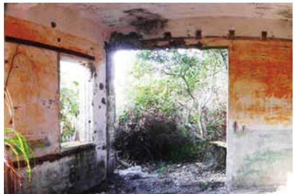
**Figure 21:** The storage room with large sliding steel door to the open space in the front. Note the wall was painted in different colours different colours at different heights for reasons yet unknown (photo by author in 2005).
