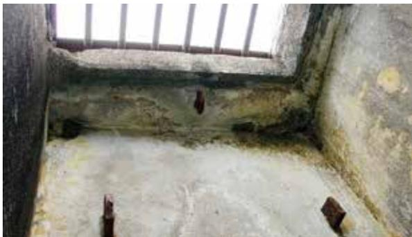
**Figure 27:** The escape shaft for the Shing Mun AOP. The two metallic remains below were for mounting a ladder. The metallic part on the roof was used to lock the steel exit door (photo by author in 2007).
