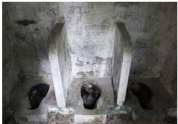
Figure 19: The "common toilet" with three squat pans separated by two short walls. Two ventilation holes on the roof maintained airflow (photo by author, 2015).
