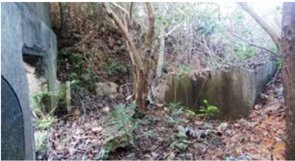
**Figure 48:** An L-shaped support wall was found outside the right-hand, lower level window. The upper section of the wall was demolished. A trench connected to the lower level window on each side (photo by author in 2016).
