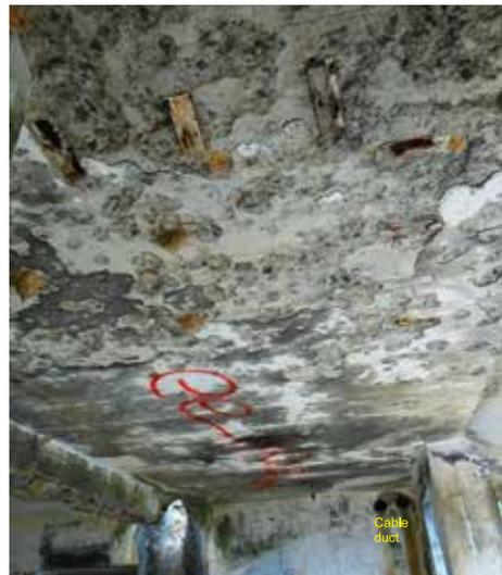
**Figure 30:** Wooden blocks laid inside the Shing Mun AOP roof used for holding cables to different observation positions via cable ducts. Note the battle damage on the surface of the roof (photo by author in 2015).
