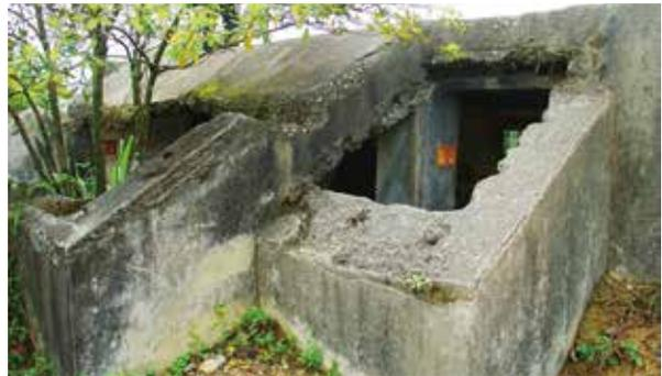
**Figure 24:** Front of the Shing Mun AOP. The small slit was for a field artillery telescope. The large opening in the back was for the DPF. Both openings had steel shutters for protection. They were removed by scavengers after the war (photo by author in 2007).
