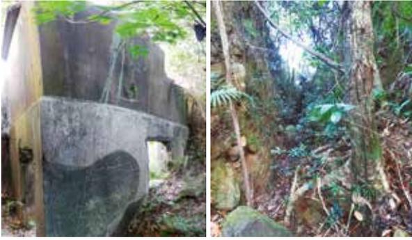
**Figure 47:** The right side of the Ping Tok Hang Shan AOP with the upper and lower entrances at the rear. The earth outside was piled up to the same level as the lower level window on one side and to the upper level in the front. The right photo shows the narrow and deep main entry trench now blocked by vegetation (photo by author in 2016).
