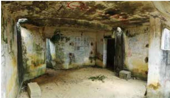
**Figure 26:** The rear of the Shing Mun AOP. The holes on the wall were for mounting three bunk beds. The openings on the left and middle were for a field artillery scope. The opening on the right led to the communication and living area. Note the support beam on the roof (photo by author in 2014).
