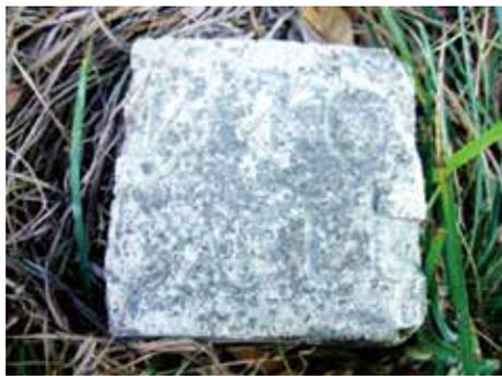
**Figure 2:** WD cable marker stone on Shatin Pass Road showing the military communication cable below (photo by author, 2009).
