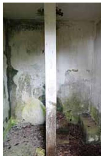
**Figure 15:** A wall dividing a toilet room into two stalls – one with a concrete stand and one without. Such a design might have been to divide users' lavatory activities. Note the lack of an open hole in the ground, as all solid waste was stored in "honey buckets" and disposed of elsewhere every day (photo by author, 2000s).
