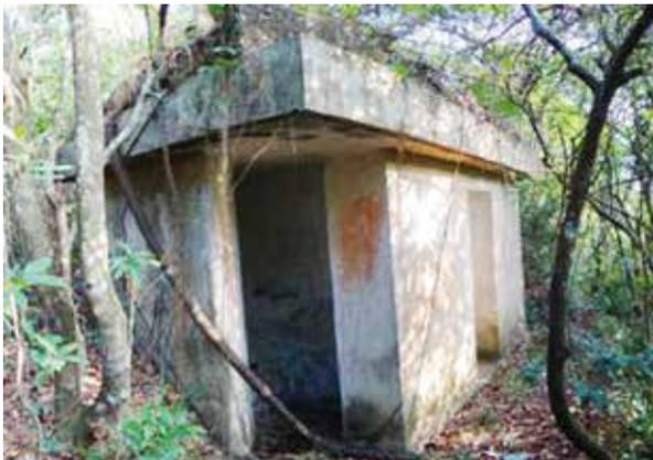
Figure 17: A pit toilet at the Tai Tam Gauge Basin Battery. The officer's toilet is in front. Note the thickness of its shelter wall (photo by author, 2015).
