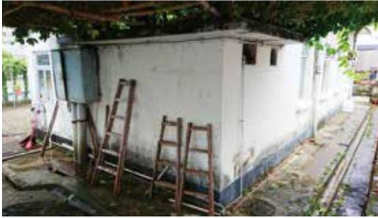
**Figure 57:** Personnel entrance side of the store room. The extended structure in front was the toilet and water tank. The square mark above the ground now blocked was for access to the toilet. All power and water pipes are modern enhancements (photo by author in 2019).
