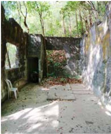
**Figure 81:** Inside of engine room with the platform for the engine and generator. Damage on top of the wall caused by removal of the roof supporting beams (photo by author in 2019).
