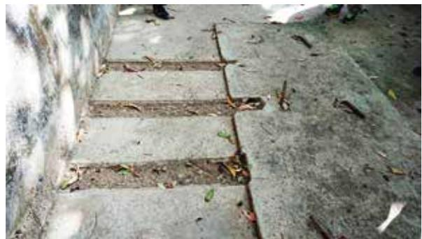
**Figure 26:** Concrete platform on floor used to install the engine and generator. Three trenches on ground used to place cables from the generator. Note the remains of large bolts used to install the engine (photo by author in 2019).
