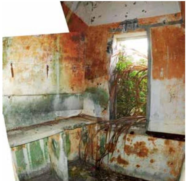
**Figure 20:** The office with a concrete table and a two-level rack mounted on the wall (both gone). Note the rail on the wall for window's sliding steel shutters (photo by author in 2005).
