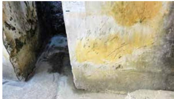
**Figure 29:** Battle damage on the Shing Mun AOP inside walls caused by Japanese hand grenades dropped from the open observation roof opening (photo by author in 2011).
