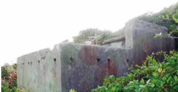
**Figure 36:** The front of the Tai Leng Tung AOP's upper level. The metal remains on its wall were racks used to hold the steel shutters for the window. Note the remains of the camouflage painted on the wall (photo by author in 2016).
