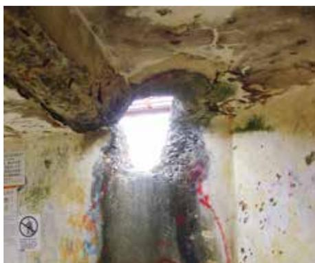
**Figure 33:** Damage on the Shing Mun AOP roof caused by scavengers removing large steel reinforcement bars below the support beam. The shape of the removed rebars is still visible on the damaged surface (photo by author in 2007).
