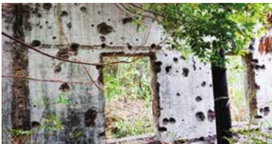
**Figure 32:** Splinter damage on the inside wall (photo by author in 2019).
