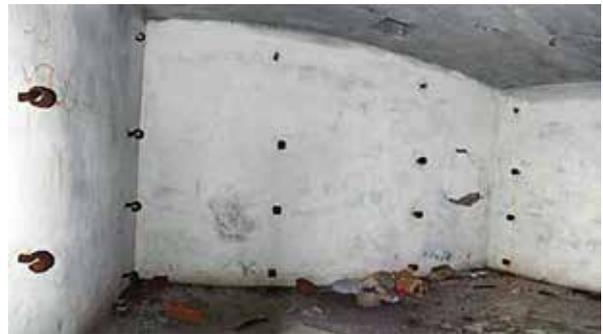
Figure 9: Inside a shelter. The metal rings on the wall were used to mount foldable beds. Three bunk beds were mounted on each wall in this shelter. Note the square-shaped ventilation hole on the roof (photo by author, 2016).
