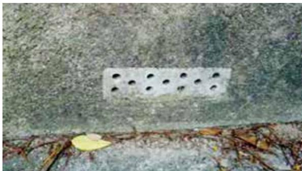
**Figure 12:** Ventilation holes along the front wall of the shelter (photo by author, 2007).
