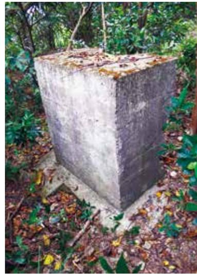
**Figure 78:** Rear of power terminal box. The underground cable duct connected to the box on the left side of photo (photo by author in 2014).
