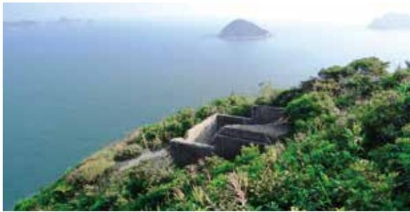
**Figure 35:** Tai Leng Tung AOP with Steep Island in the background. The roof and upper level floor was demolished after the war to prevent the structure from being occupied by squatters (photo by author in 2016).
