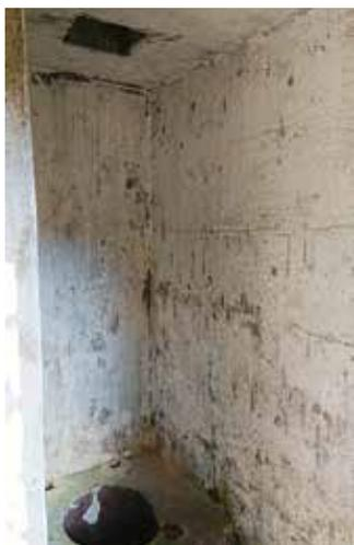
Figure 18: The "executive toilet". Note the toilet seat inside and ventilation hole on the roof. A wooden plate served as a toilet seat on top of a concrete step. A hole on the wall was possibly used as a toilet paper mount (photo by author, 2019).
