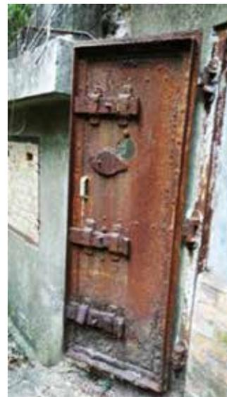
Figure 10: Heavy steel door for the shelter. Note the three huge locks inside the door. The hole on the door allowed the occupants to shoot out from behind the door. The hole could be covered by a steel plate when not in use (photo by author, 2016).
