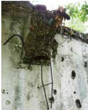
**Figure 36:** Damaged supporting beam with rebar (photo by author in 2019).
