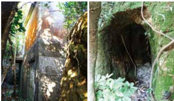
**Figure 37:** The rear of the Tai Leng Tung AOP entrance hidden inside a large cave. Two trenches on the ground connected to the upper and lower entrances. A steel ladder would have been installed on the platform outside the upper entrance to facilitate access. Note a T-shaped Japanese tunnel dug inside the hill behind the AOP (photo by author in 2016).
