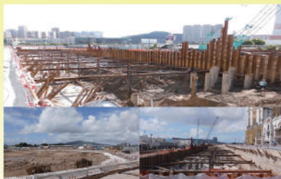
Basement & Sub-structure - Galaxy Macau Phase 2 (2016)
