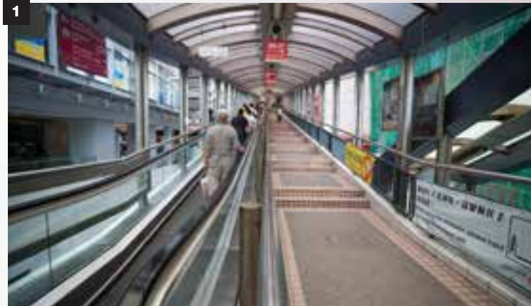
1. Current view of CML Escalator System.
