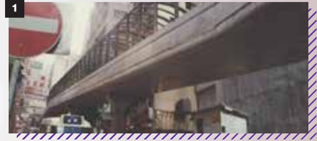
1. Central-Mid-Levels Escalator System under construction.
