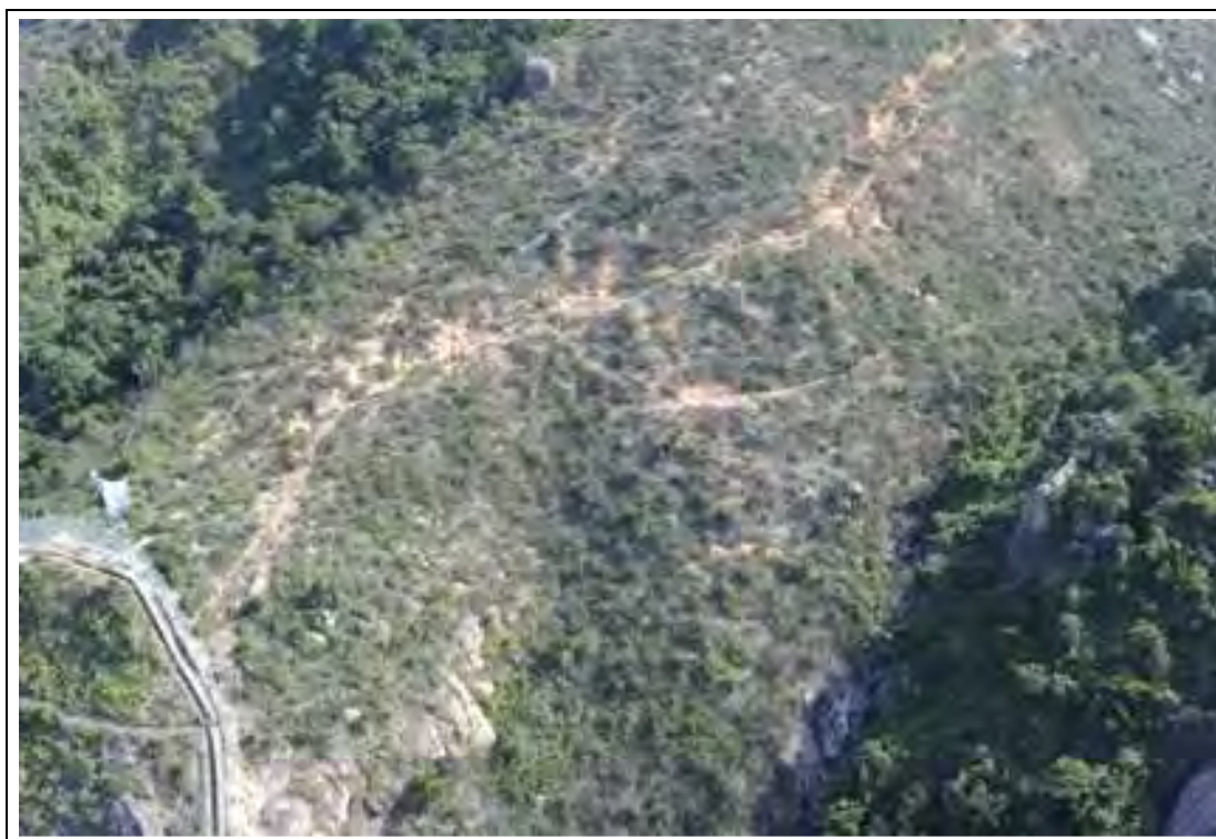
Figure 5.1. The appearance of the subject hillside of the project
