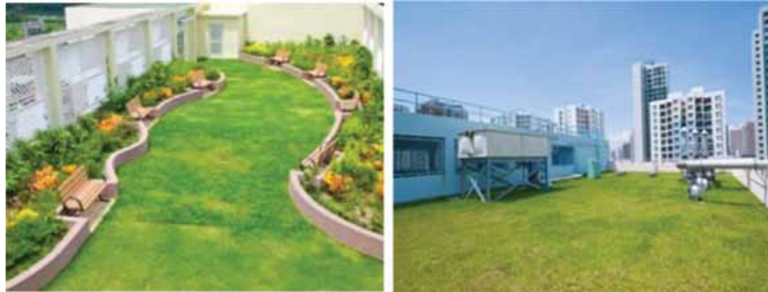
Figure 6.4 Intensive (Left) and Extensive (Right) Green Roof Garden
