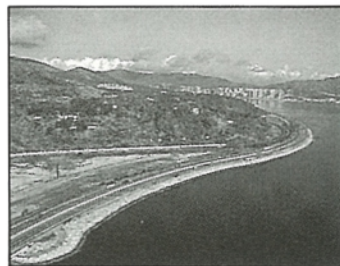
Tolo Highway — Seawall Construction
