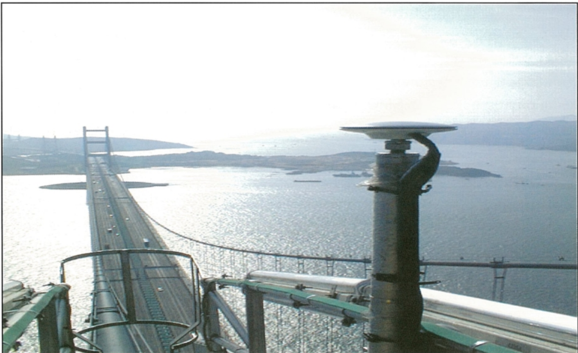
Figure 3: Tsing Ma Bridge Monitoring by GPS
