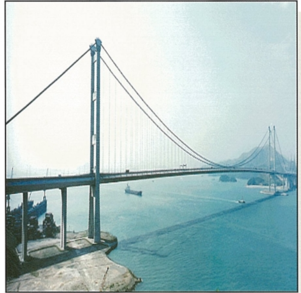
Tsing Ma Bridge from a Vantage Point, Looking West Towards Ma Wan
