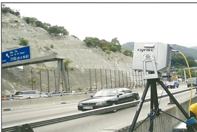
Figure 5: Application of 3-D Laser Scanning in Slope Survey
