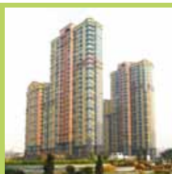
Property Development Shijiazhuang "Arc de Royal" - Phase 2
