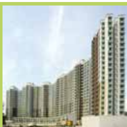
Buildings Carcass Works Contracts for Proposed Residential Development at Hung Shui Kiu, Yuen Long Lot 2064 in DD 121
