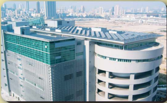
Electrical & Mechanical Services Department New Headquarters at Kai Tak Steel Roof Structure with Aluminium Roofing System (13,000 m 2 )
