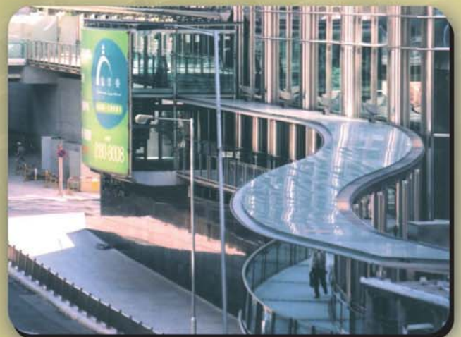
S-shape Steel Footbridge at Cheung Kong Centre Footbridge (130m in length) formed by tailor-made high strength structural steel members
