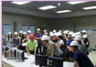
Study Tour 2014 - Pump Station Control Room
