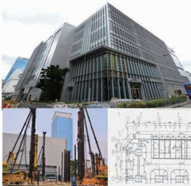
MTRC PROJECT - NEW INTERNATIONAL MAIL CENTRE (SHATIN TO CENTRAL LINK)
