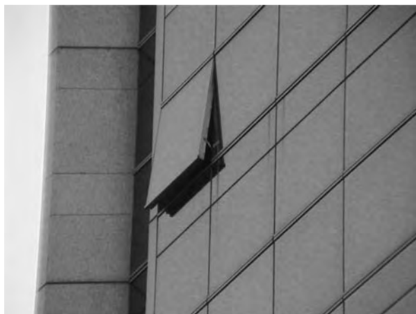
Figure 7: Sha Tin Government Offices Building
