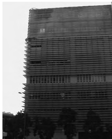
Figure 9: New EMSD Headquarters
