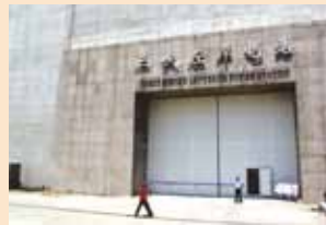
The entrance to the Left Bank Three Gorges Power Station
