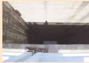
The deep hole of the spillway steel gate
