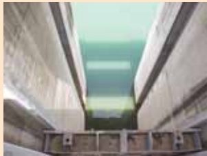
Inner part of the spillway
