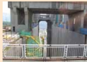
The ship lift under construction from the rear.
