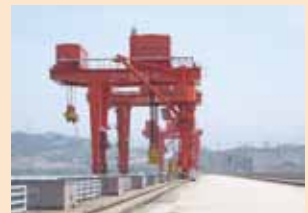
The Gantry Crane for lifting the water-stop gates of spillways
