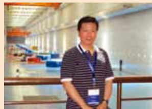
Inside the Power Plants Room
