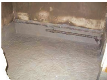
Waterproofing layer to the floor and skirting of a toilet
