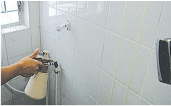
Spray deep penetrating sealer on the existing mortar pointing
