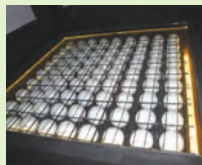
New floor slab technique – light weight concrete
