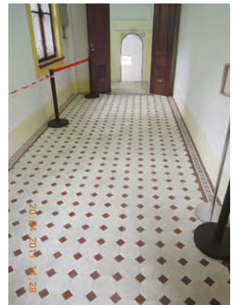
Floor Cement Tile
