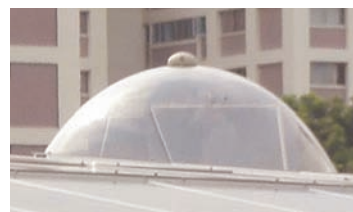
Figure 4: Light Pipes with Solar Tracking Device
