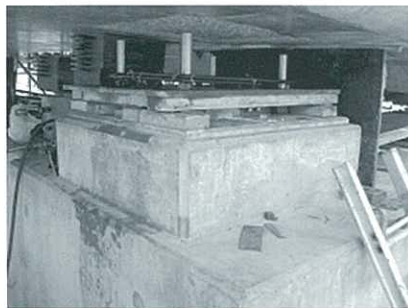
Bearing - Before Grouting
