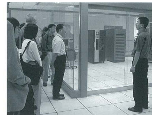
The officer in charge of Shaanxi Bureau of Surveying and Mapping introducing the mainframe of the data storage.
