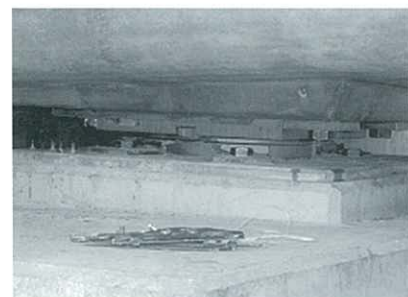
Bearing - After Grouting
